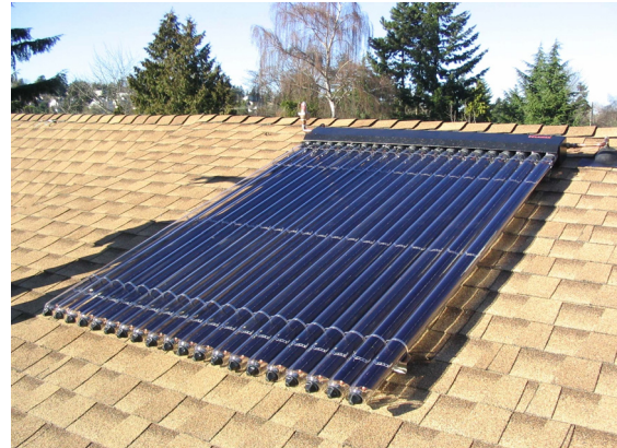
(Left) This Built Green home has a 3kW photovoltaic array that returns electricity to the power grid. (Blip Design Architects of Seattle); (Right) A solar hot water collector on the roof of a Seattle Built Green home heats most of the domestic hot water for residents. (Sunshine Construction )
