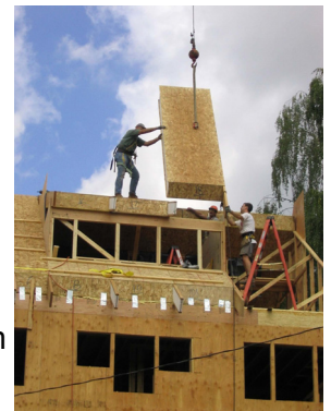
Structural Insulated Panels (SIPs) offer an air-tight construction system.
