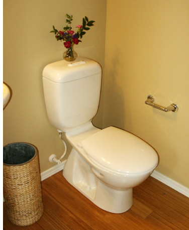
(Left) This dual flush toilet at the PSE Built Green Idea Home allows you to flush with more or less water as needed. (Right) This 'tankless' water heater by Takagi heats the water as it is needed. As well as providing hot water to fixtures and appliances, it circulates throughout the house to hydronic radiators to heat the house.
