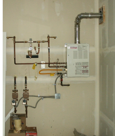
(Left) This dual flush toilet at the PSE Built Green Idea Home allows you to flush with more or less water as needed. (Right) This 'tankless' water heater by Takagi heats the water as it is needed. As well as providing hot water to fixtures and appliances, it circulates throughout the house to hydronic radiators to heat the house.
