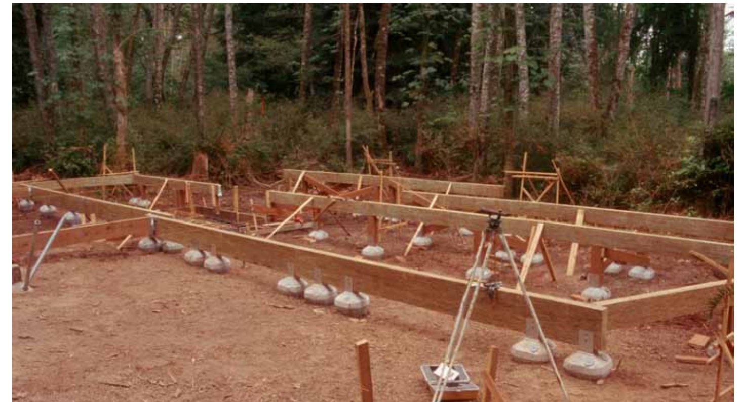
Low impact foundation systems require minimal excavation, reducing site impact and maintaining a site's natural hydrology. They also reduce the amount of concrete needed for foundation work, and can virtually eliminate the need for formwork—reducing materials use and associated resource extraction and energy impacts.
