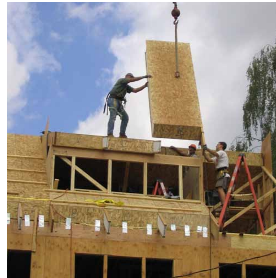
Structural insulated panel roofs eliminate installation problems that can result in roofs and walls performing at lower than specified thermal values.
