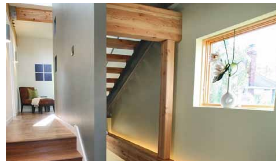
Operable windows for cross ventilation are part of a larger strategy of natural ventilation which can include open-plan spaces and open stairwells for air movement.
