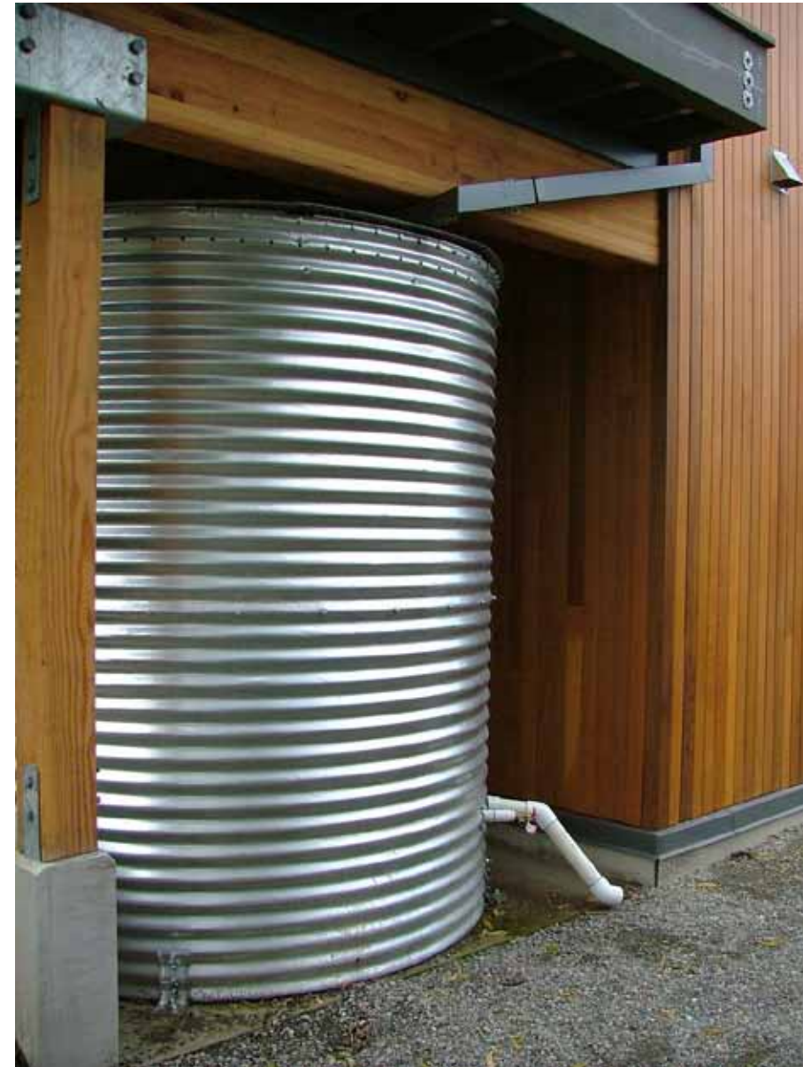
Cisterns can take a variety of forms, and can be installed above-grade, below ground, or partially buried. This steel cistern is placed under a porch. Above ground systems can sometimes utilize gravity for water distribution, eliminating the need for pumps.
