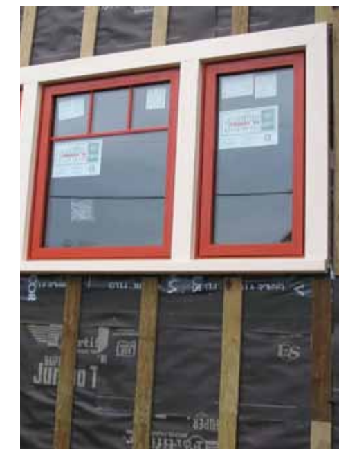
The rain screen approach allows for a wide variety of siding applications, from modern to traditional.
